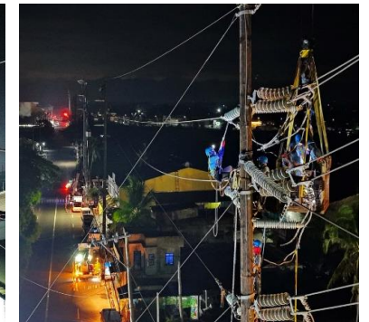
Uprating of Portion of Dila-Real 115 kV Line
