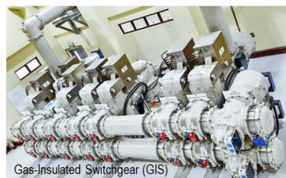
Gas-Insulated Switchgear
