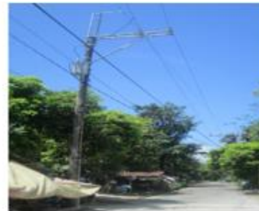
Completed line works at Brgy. Caralao, Majayjay, Laguna
