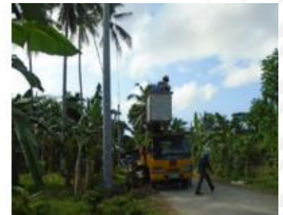
Line works at Sitio Pitogo, Binahaan , Pagbilao, Quezon
