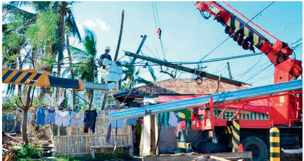
(Above) Meralco's South Distribution Services personnel clear a fallen electric post on a roof of a damaged house in Roxas City, Capiz. About 90 percent of electric facilities in the province were damaged after Yolanda hit the province. (Middle) Meralco's "Panay Contingent" line up along Aklan West Road on their way to their respective assignments in Aklan, Capiz, and Iloilo. The contingent is composed of 16 vehicles/equipment with 61 personnel assigned to assist the electric cooperatives in these provinces. (Below) Meralco Central Distribution Services personnel erect power poles in Kalibo, Aklan. (Photos courtesy OMF)
