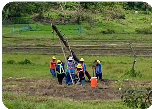
Meralco linemen helped restore power in several towns of Ilocos Norte—Paoay, Laoag City, Bacarra, Pasuquin, and Dingras—severely affected by super typhoon Egay. By immediately restoring power, they contributed to bringing back normalcy in the areas the soonest possible time.
