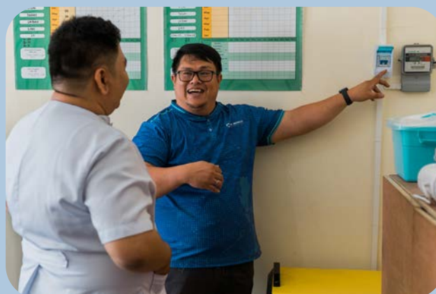
Barangay health workers and personnel are trained on how to use and maintain the solar PV system powering their health center.
