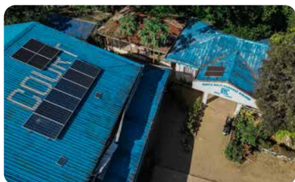
The health station in Barangay Laiban is more equipped to handle basic services with the help of solar power.
