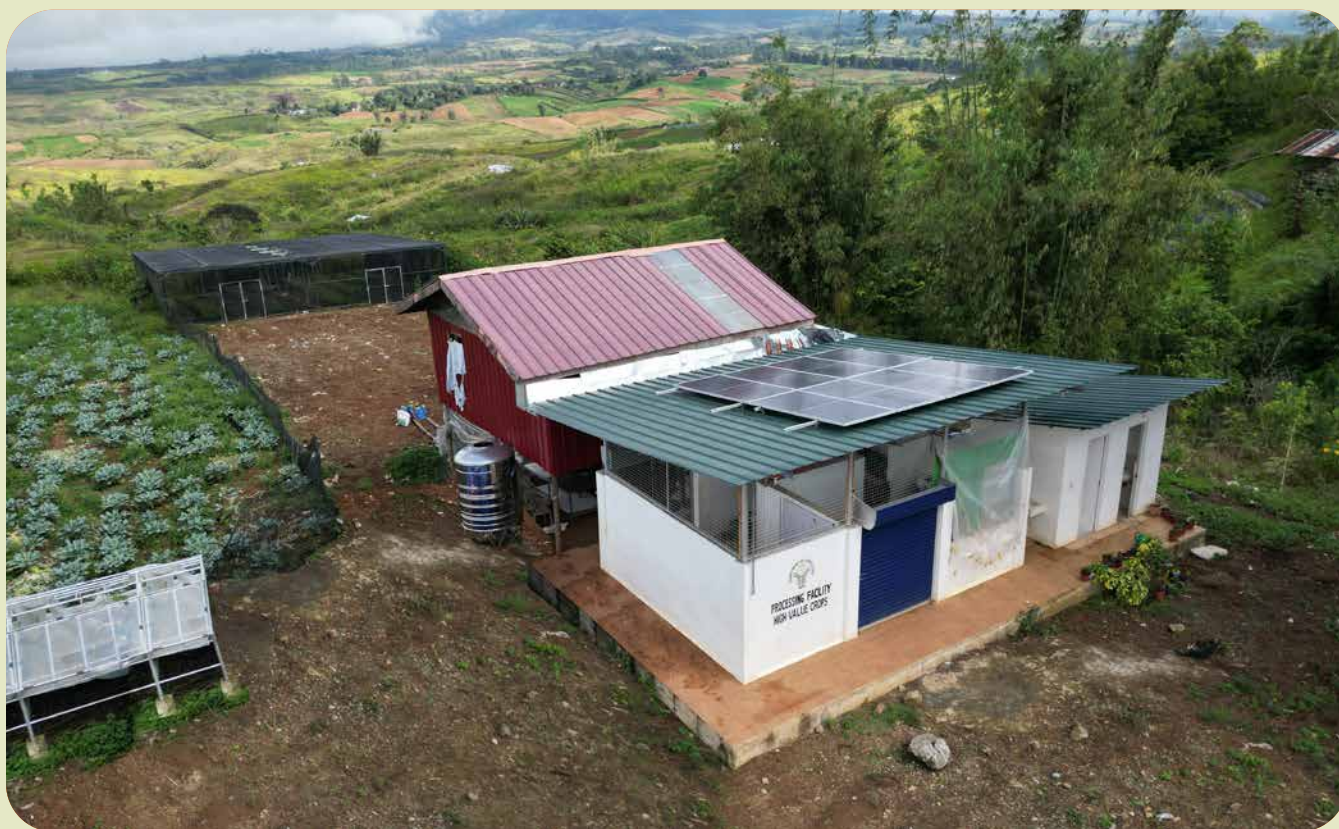
Work is faster and more efficient at the MILFACO livelihood facility now that it is energized.
