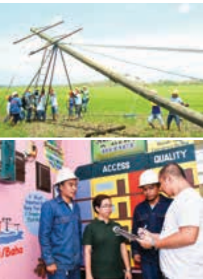
Top: Meralco linemen and engineers manually erect a downed pole in Aparri, Cagayan during a power restoration activity in the aftermath of Typhoon Ompong (international name: Mangkhut). Since the pole was located along a rice paddy, heavy lifting equipment could not be used due to the unstable soil. By the end of the project, the 66-member crew successfully rehabilitated the 69kV Magapit-Zatinga-Lucban backbone serving two substations of CAGELCO II.
