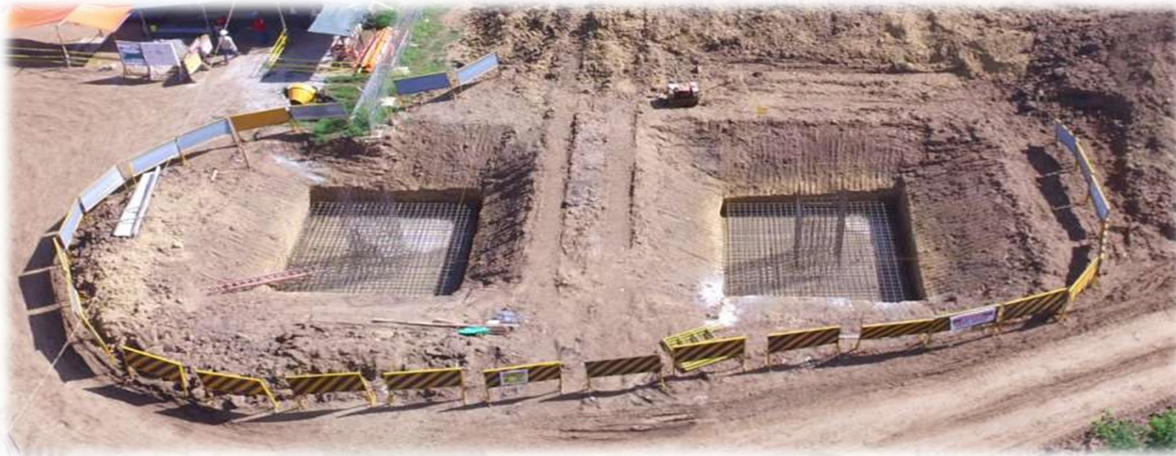
Pad and Chimney Foundation for Self-Supporting Steel Poles 1 and 2
