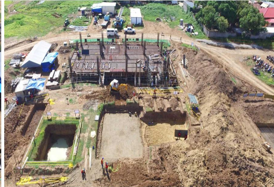
Main Transformer and Capacitor Bank Foundation Excavations
