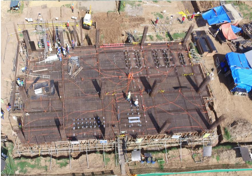
Main Control Building Foundation Works
