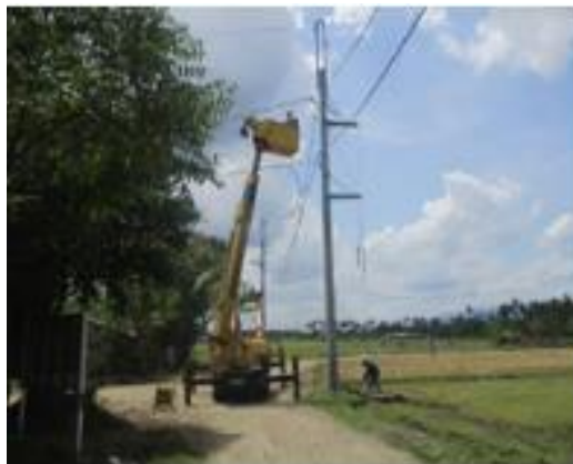
Line works at Brgy. Del Valle , San Antonio, Quezon
