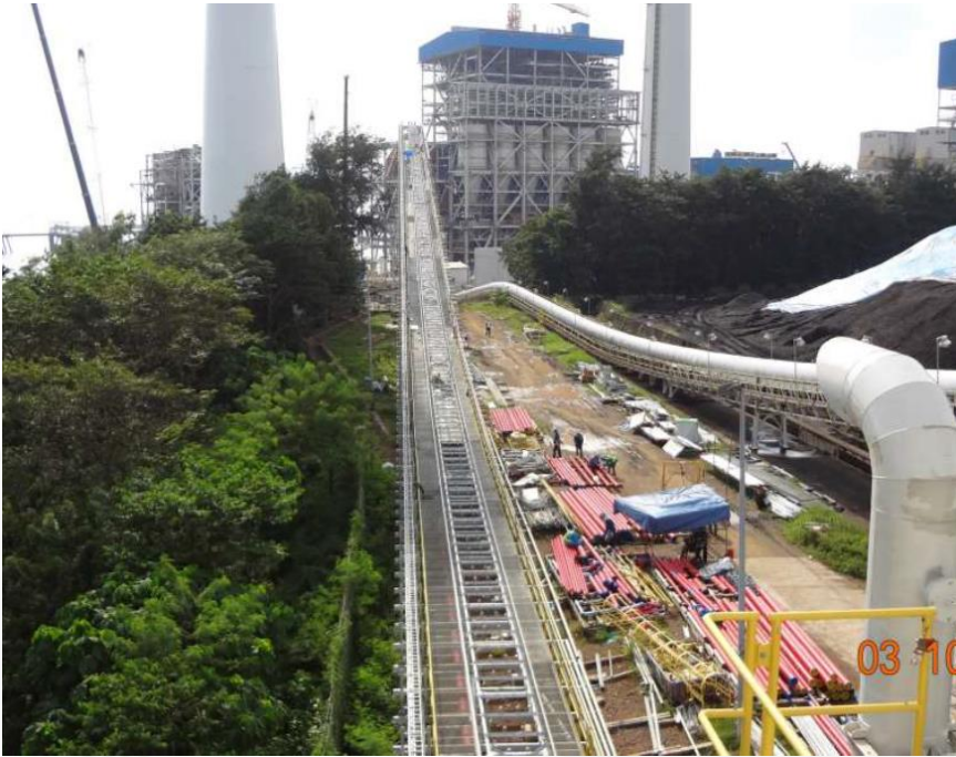
Boiler Building and Coal Conveyor
