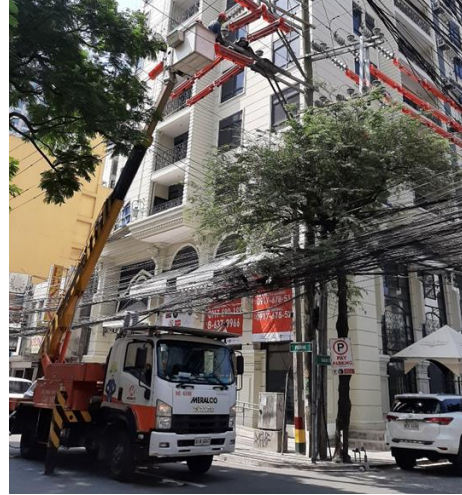
Replacement of Insulators
