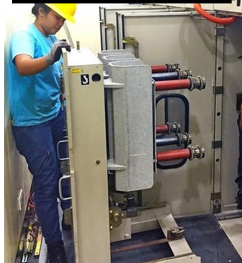
PMT of Power Transformer Bank
