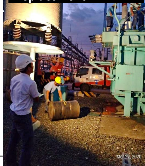
115 kV HO Bushing Replacement
