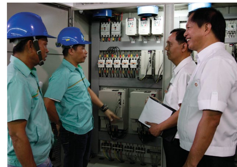
Meralco Technical Services Engineer Dean Sempio and Relationship Manager Rolan Mercado (third and fourth from left) are joined by Saffron Philippines Electrical Section Supervisor Ricardo Pacomio and Assistant Supervisor Teodoro Macugay (second and far left) as they inspect the plant’s electrical facilities.
