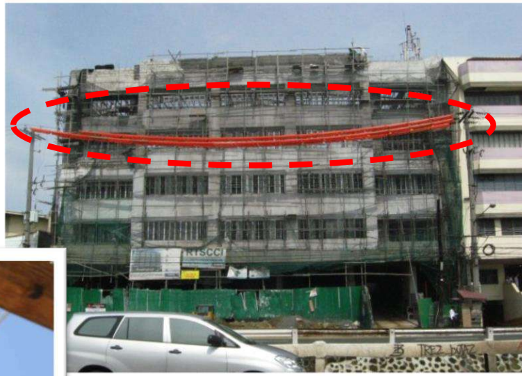
Installation of conductor covers to provide barrier to construction workers.
