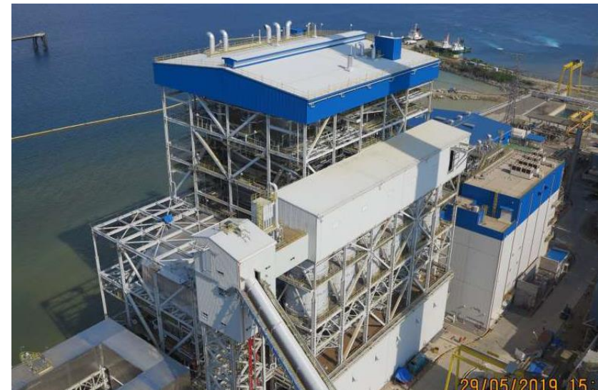
Boiler, Pulverizer, and Main Control Building
