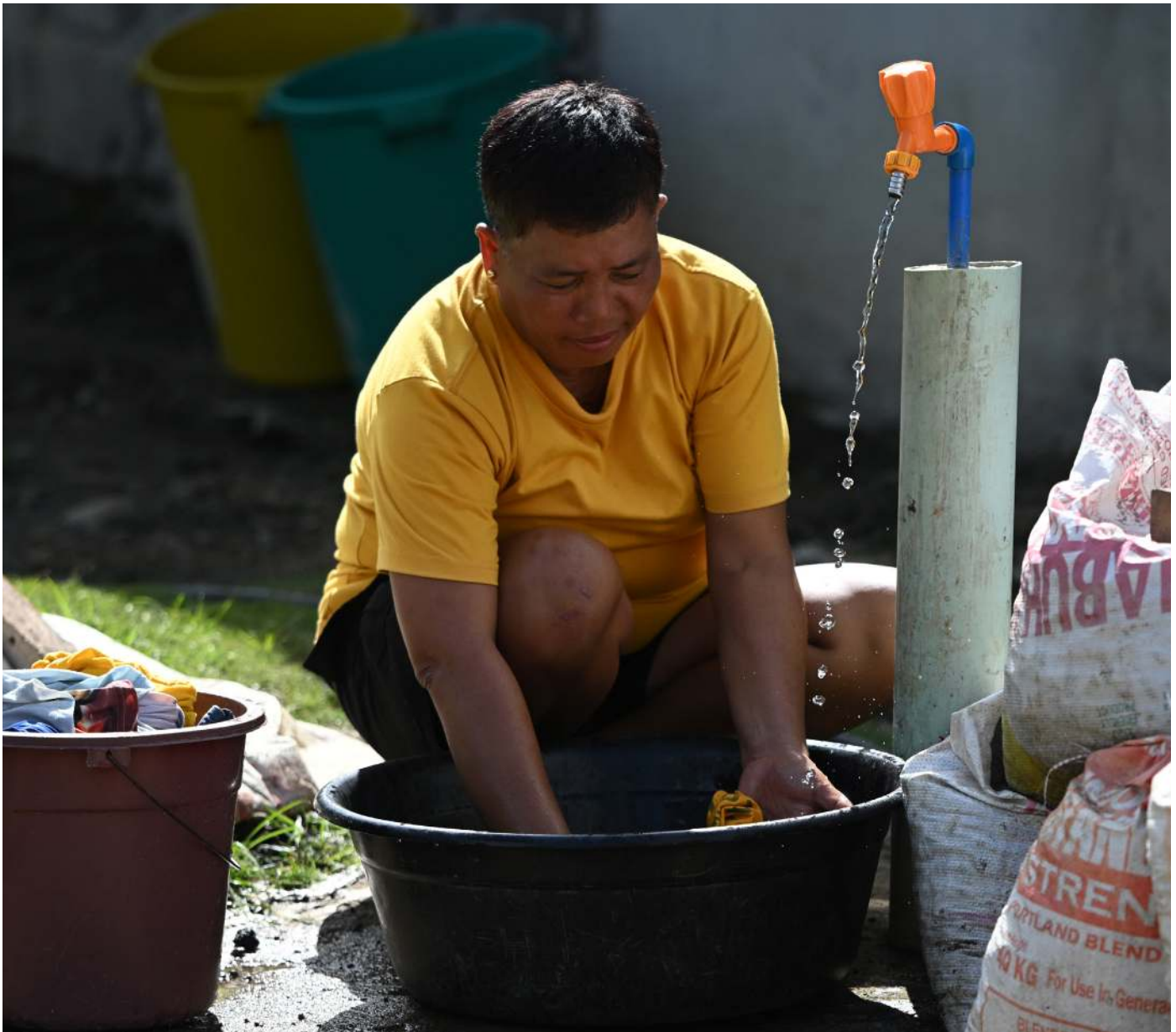
Corina Pamplona no longer needed to bring her family's laundry to the deep well. With a solar PV system powering their water access facility, clean water is now accessible closer to home through communal taps.
