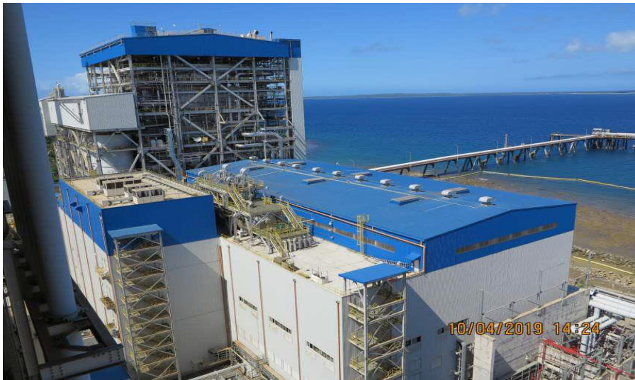
Boiler, Steam Turbine Generator (STG) Building and Main Control Building
