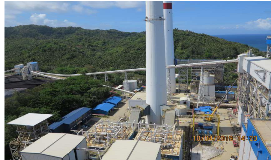
Coal Transfer Tower 1 & 2 and Coal Conveyor
